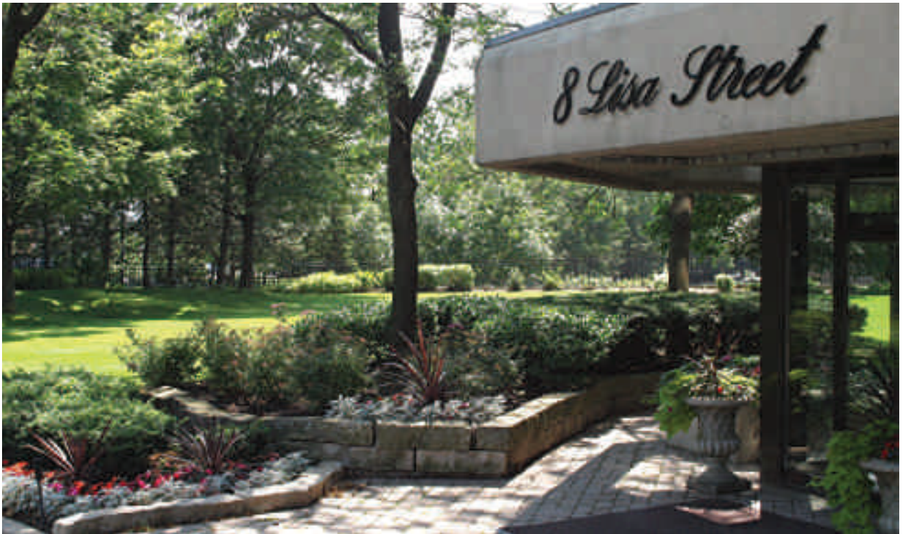
The Ritz Towers, PCC 260, completed a series of infrastructure projects in less than four years.
